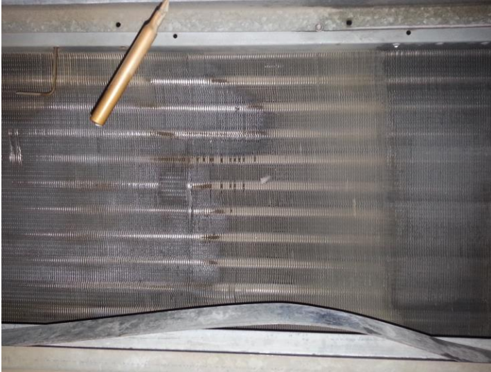
Above is a before and after look at the coils in the main AHU at [redacted]. Below is a look at the condenser coil on the unit to the right during cleaning.
