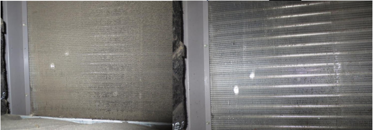
Above is a before and after look at the coils inside the access panel we cut. Below is a look at the coil during the cleaning.
