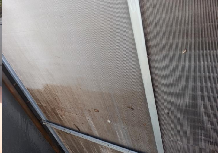
Above is a before and after look at the coils in the main AHU at [redacted]. Below is a look at the condenser coil on the unit to the right during cleaning.
