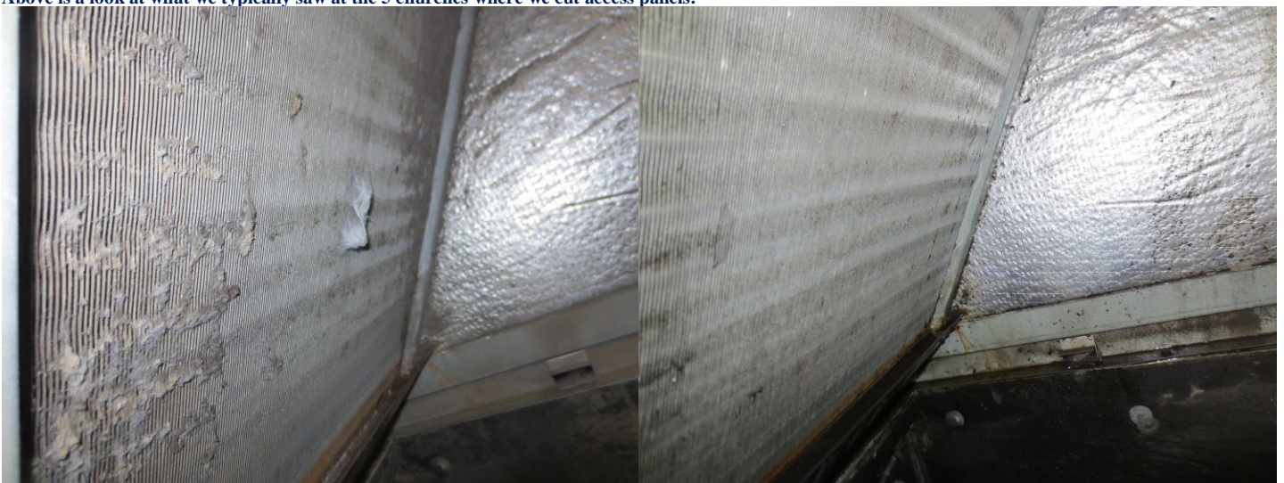
This is a before and after look at a unit at [REDACTED]. These units were really dirty and saw some oxidation exposed after the cleaning.
