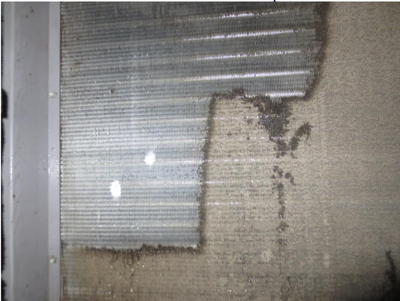
Above is a before and after look at the coils inside the access panel we cut. Below is a look at the coil during the cleaning.
