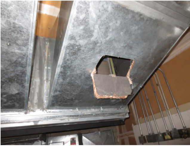
This is the access panel cut into the AHU @
